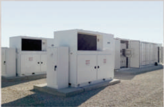
40HC 800KW/524KWH Lithium-Ion Battery
